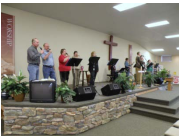
The Brick around the stage is being completed
